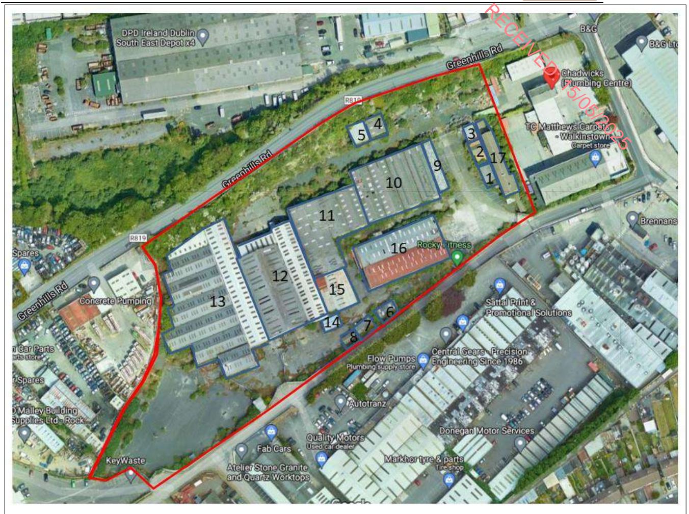
Figure 3 Buildings grouped and numbered 1 to 17. Plates in Appendix A show the groupings
