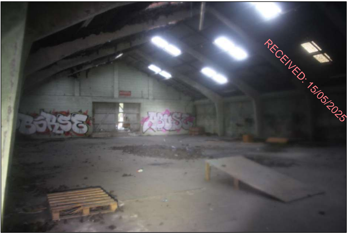
Plate 14 Building 12 – Low Bat Potential (October 2023)
